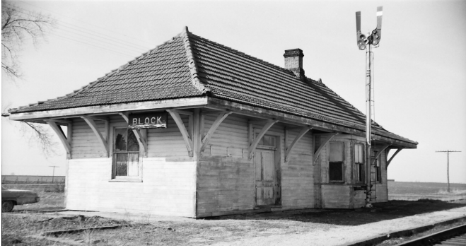
Block Station, Block IL
